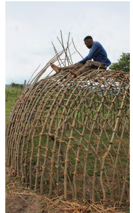
Thin poles used for roof construction which supports thatch grass. (Photo: Shannon Herd-Hoare)
